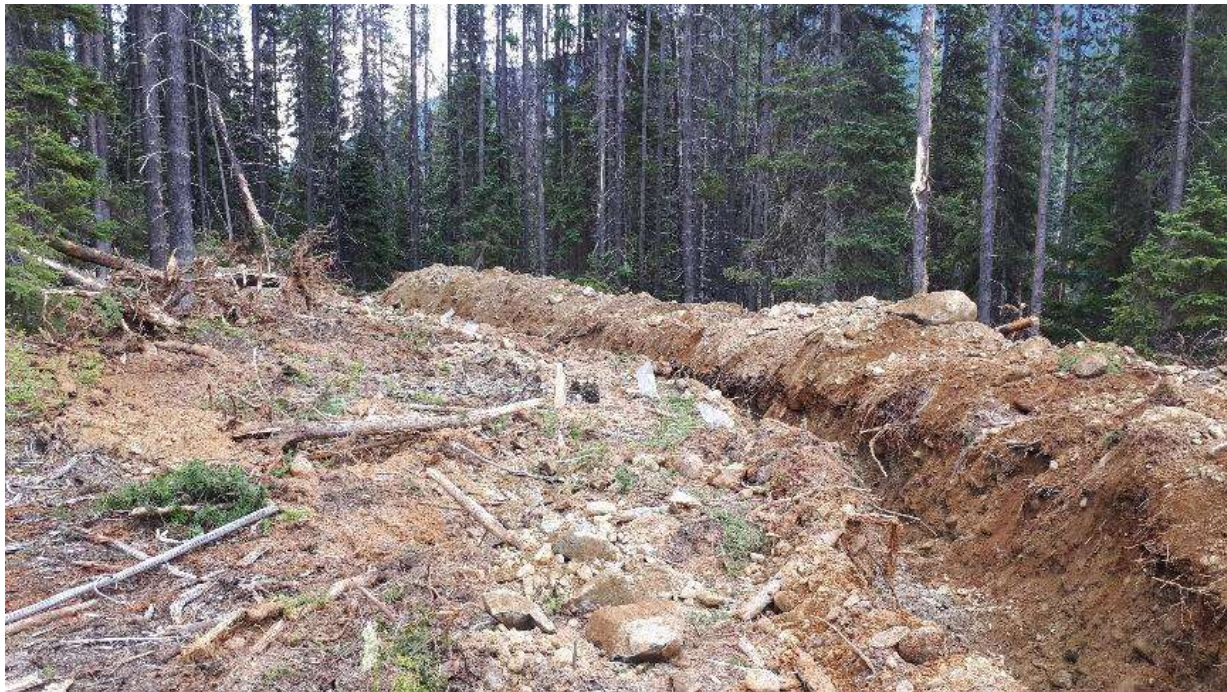
Photos of new trench at Lucky Todd
