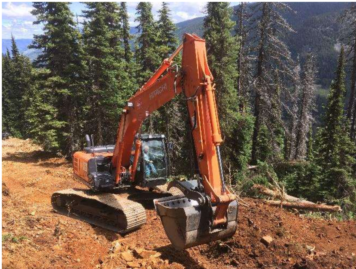
Access road construction
